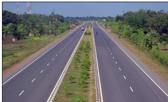
FIGURE 15-4 STRENGTHENING OF THE NH 530B ROAD
